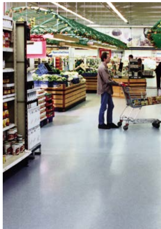
MMA floor coating in a supermarket
