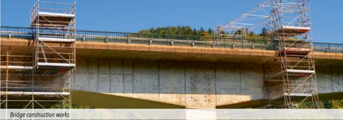
Bridge construction works
