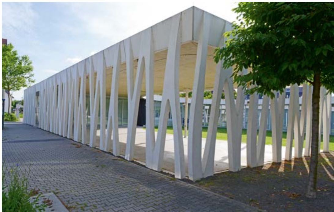
Self-compacting concrete, Community Centre Mannheim
