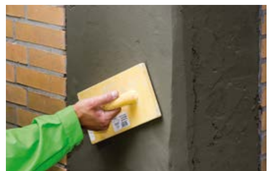
Application of repair mortar
