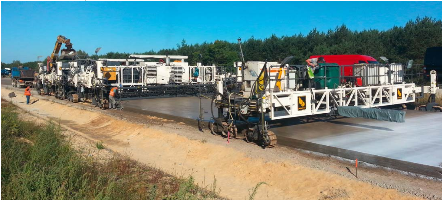
Illustration 1: Towed stage unit
